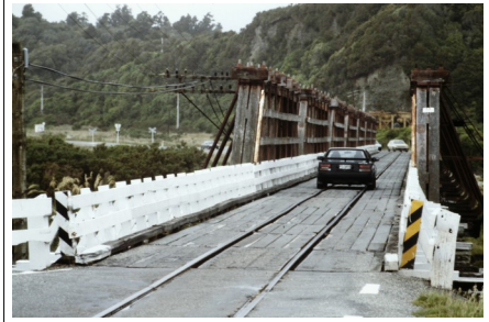
DUAL PURPOSE CAR & RAILWAY BRIDGE (NEAR GREYMOUTH)
